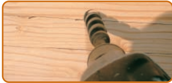
Drilling holes in glulam is permissible if done properly. (See below for details.)
